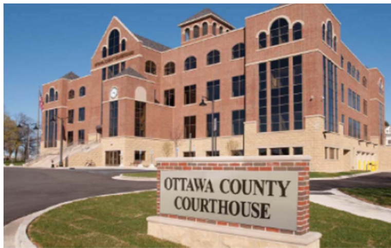
Facilities and Maintenance is responsible for eleven County facilities. The Grand Haven Courthouse, pictured above, is the newest facility which opened in 2009.
