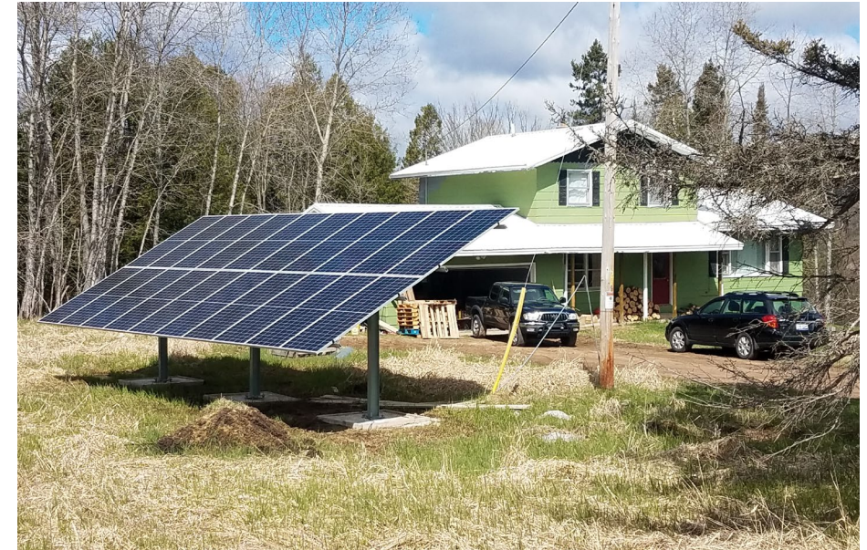
Rock River Township; Brad Neumann
