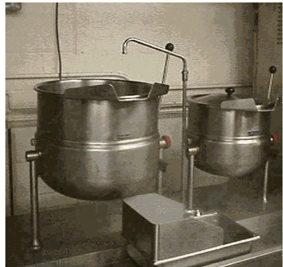
Water Fill to Steam Kettle
