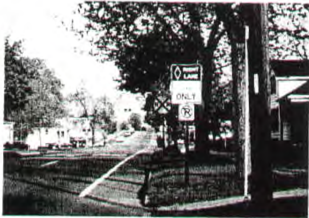
Local units of government in Ottawa County have developed bike lanes and separated pathways in communities such as Grand Haven (above), Spring Lake, Coopersville, Allendale, Hudsonville, Georgetown Township, and Holland.
