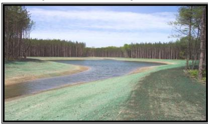
completed the construction of a clay cap over the landfill in 2008. This will prevent the contamination located in the landfill from leaching to the groundwater (via percolating rain water), and an upgrade to the purge well and treatment system began in 2008. The cost is expected to be approximately \$3.8 million with the work being completed in 2009.
