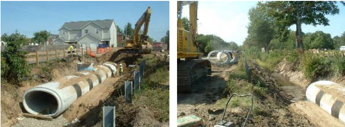
Storm sewer installation
