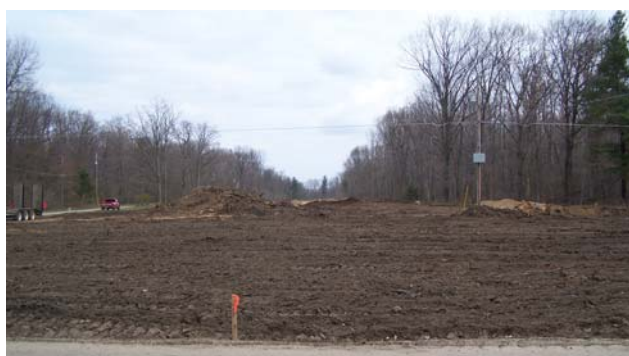
Looking north from Johnson Street at M-231 clearing
