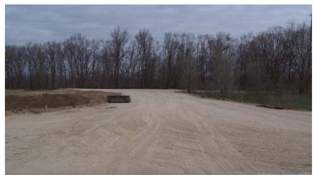
Looking north from Cedar Street at M-231 clearing
