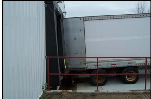
Loading Dock, after Phase 1
