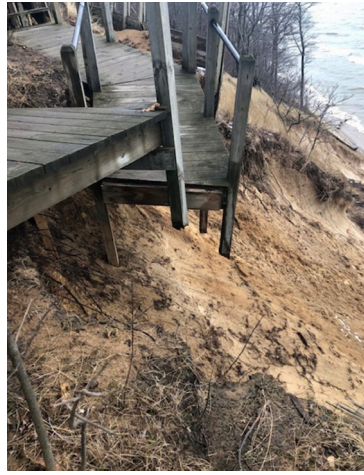
Ridge trail at Kirk Park collapsed due to erosion
