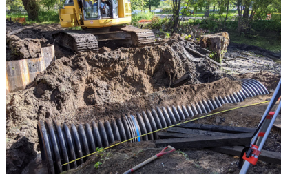
New culvert being placed under road
