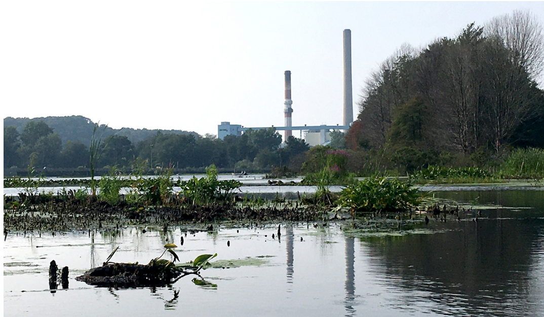
The J.H. Campbell Generating Plant as seen from the Pigeon River mouth in Port Sheldon Township. The Consumers Energy Complex is set to cease operation in 2025.
