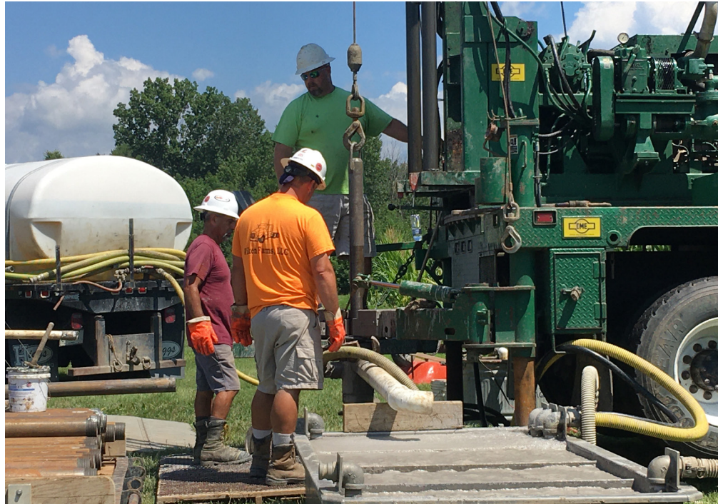
Above: Workers drill a well in Olive Township in August 2021 for the Michigan Geological Survey and Ottawa County that contains monitoring sensors that provide real-time aquifer data. Right: Former Land Use Planning Specialist James Kilborn discusses the well drilling process on location with Michigan Geological Survey Director John Yellich.
