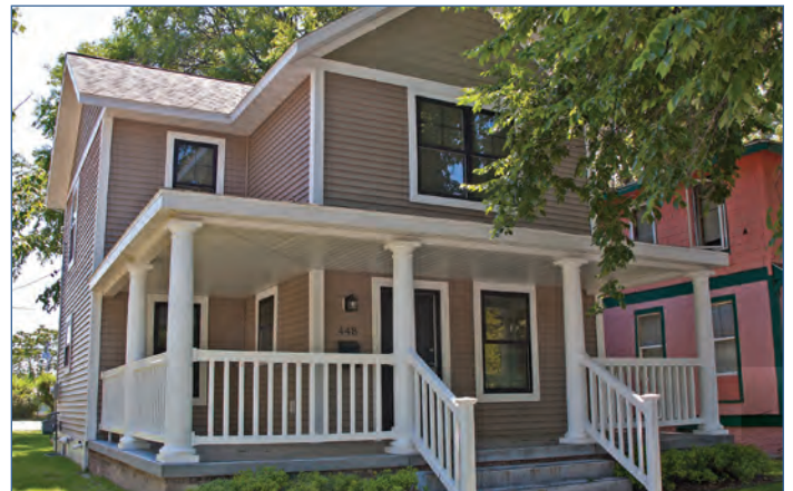
One of 15 Scattered Sites homes being renovated in preparation for sale
