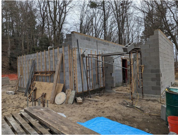
New concrete block wall in progress
