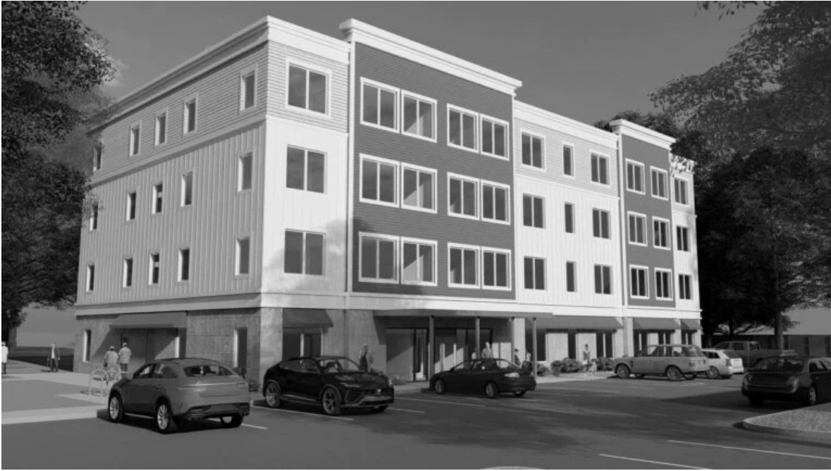
Renderings from Pinnacle Construction Group show designs for Samaritas Spring Lake at 734 E. Savidge St. in Spring Lake Township. Credit: Courtesy image
