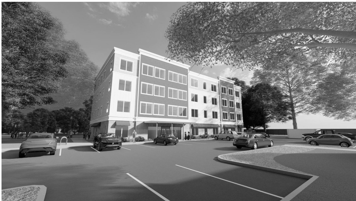
Once completed in 2025, Samaritas Spring Lake will be the first multifamily certified passive housing development in the state of Michigan. Credit: Courtesy image
