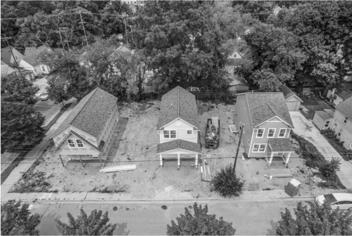
Construction on an ICCF Community Homes project in Grand Rapids' Baxter neighborhood in mid-2023. Credit: ICCF Community Homes
