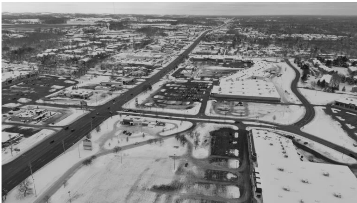
A drone shot shows the Alpine Avenue corridor in Walker from near the I-96 interchange looking north. Credit: City of Walker
