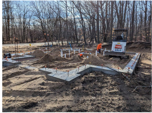
Day Use restroom foundation and utilities
