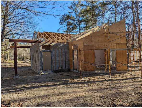
Framing and roof in progress
