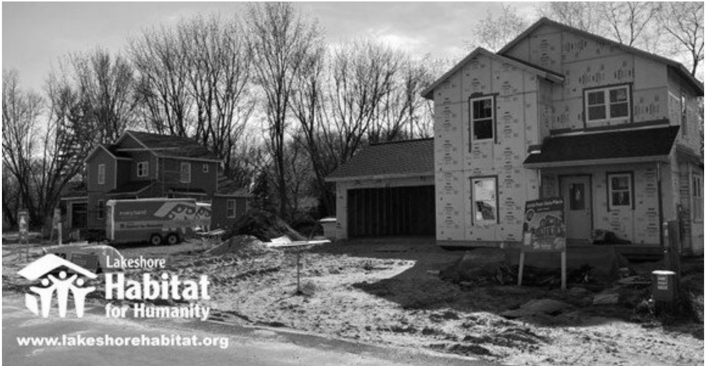
A Lakeshore Habitat for Humanity development underway near Holland.
