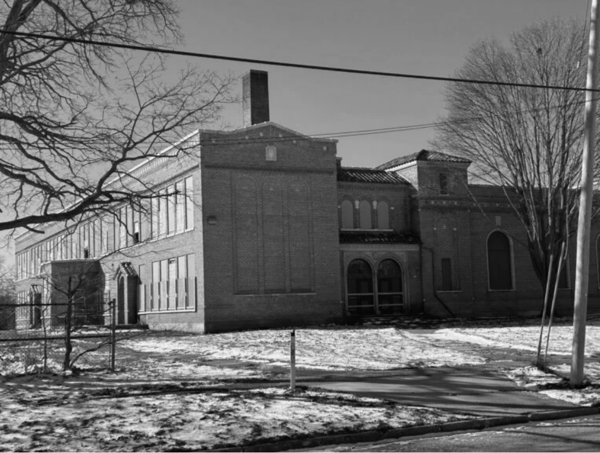
The Muskegon County Land Bank received $1.4 million to rehabilitate the 94-year-old former Froebel School in Muskegon that Samaritas plans to convert into housing. Credit: Muskegon County Land Bank Authority
