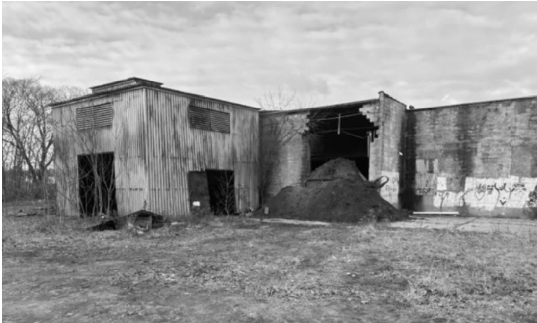
This industrial building at 1367 W. Sherman Blvd. in Roosevelt Park will be demolished with help from a $440,000 blight elimination grant to make way for future development. Credit: Muskegon County Land Bank Authority
