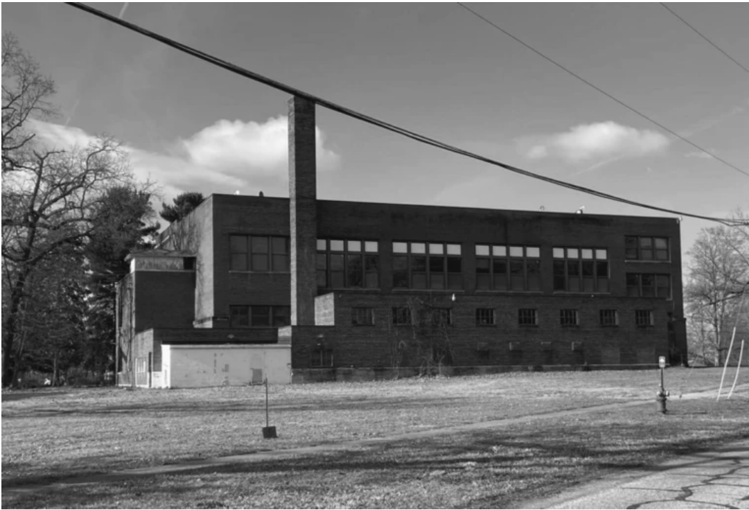
A recent grant will help restore the former Decatur High School at 312 School St., also known as the Edgar Bergen building, into a mixed-use project. Credit: Van Buren County Land Bank Authority
