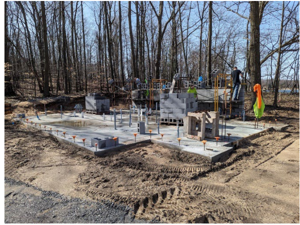
Day Use restroom masonry walls in progress
