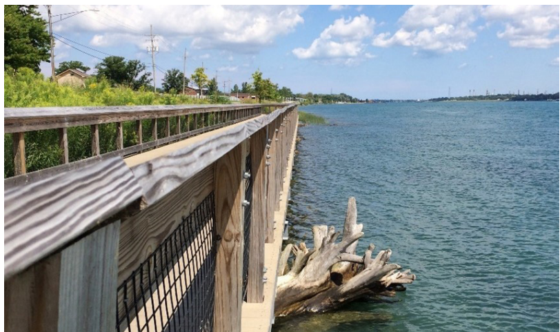
Integrated elevated boardwalk and woody habitat structures on St. Clair River, designed by GEI staff
