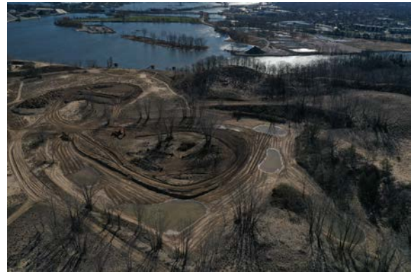
Wetland construction by GEI at OSCP
