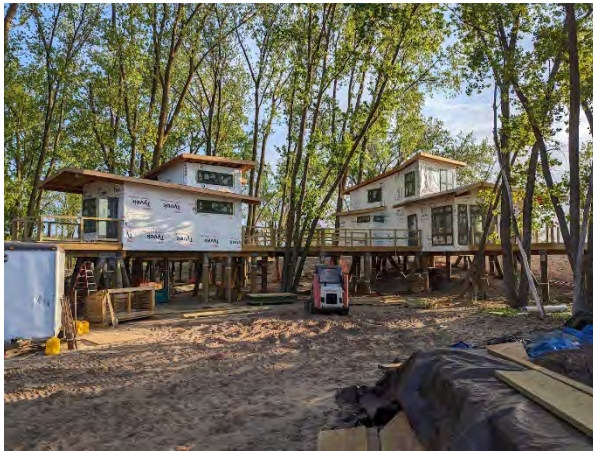
Treehouses under construction
