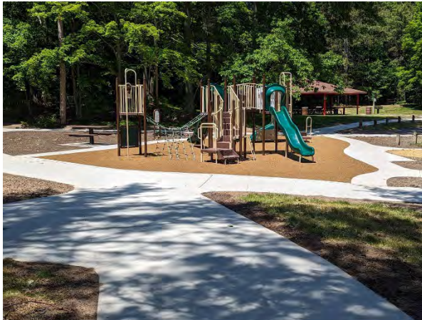
Completed playground with concrete walks
