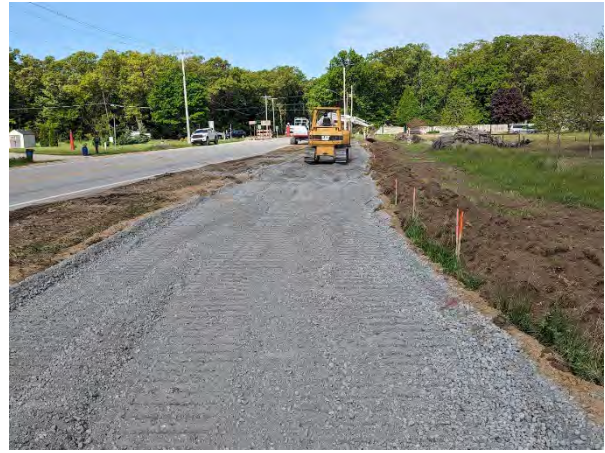
Excavation and base material near 144 th Ave.
