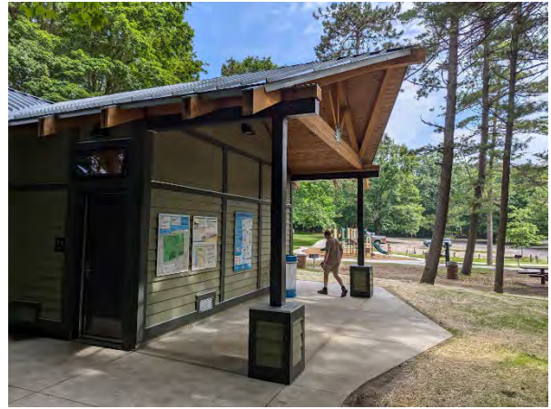
Completed restroom with trailhead maps and signage (new play area in background)
