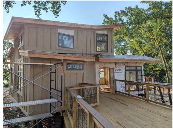
Grand Treehouse with siding in progress
