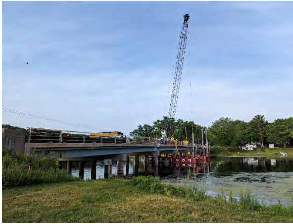
Piling installation at the Stearns Bayou Bridge
