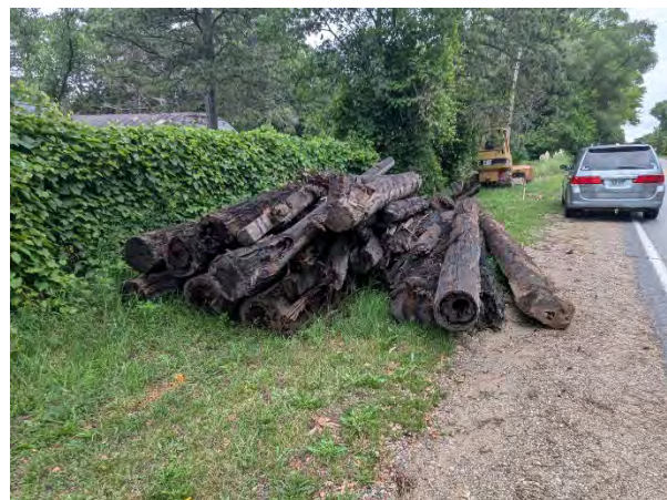
Timbers removed from piling area
