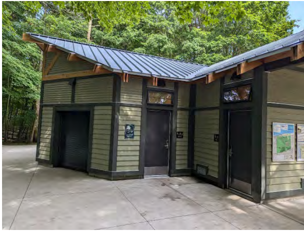
Completed restroom including grant plaque
