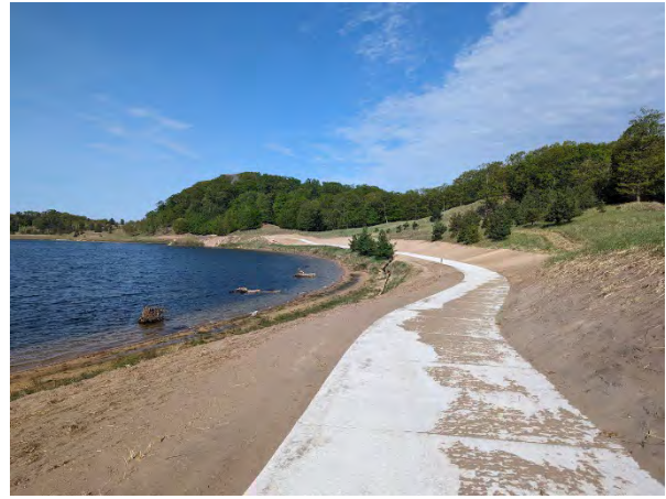
Completed lake trail loop
