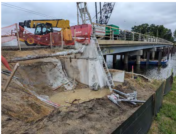
Expanded bridge abutment in progress
