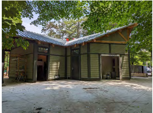
Restroom with metal roof nearing completion
