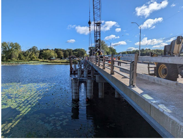
Support columns in progress
