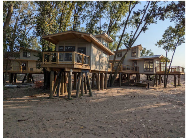
Treehouses with exteriors mostly completed
