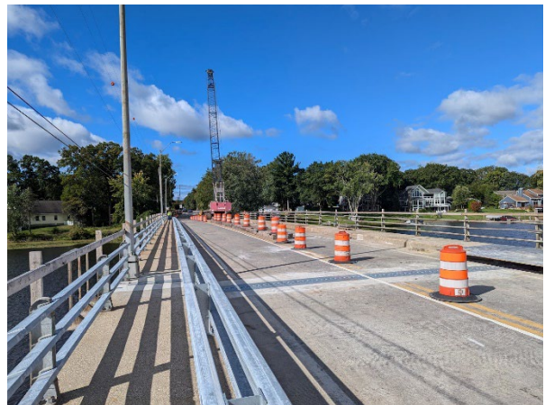
South bridge lane open looking west
