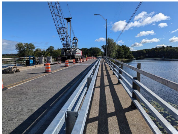
South bridge lane open looking east
