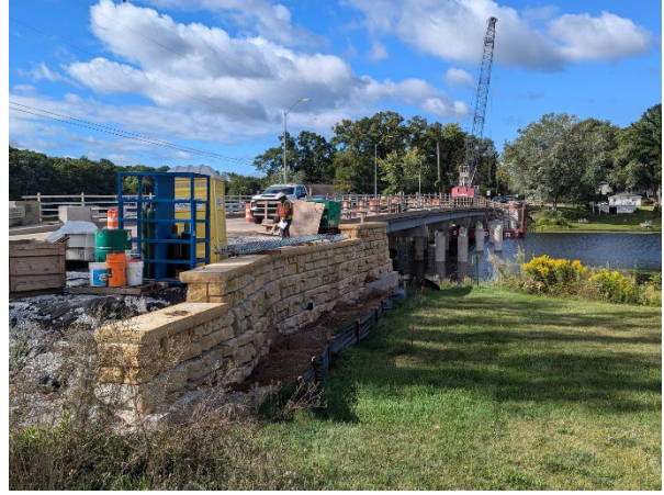
New bridge approach
