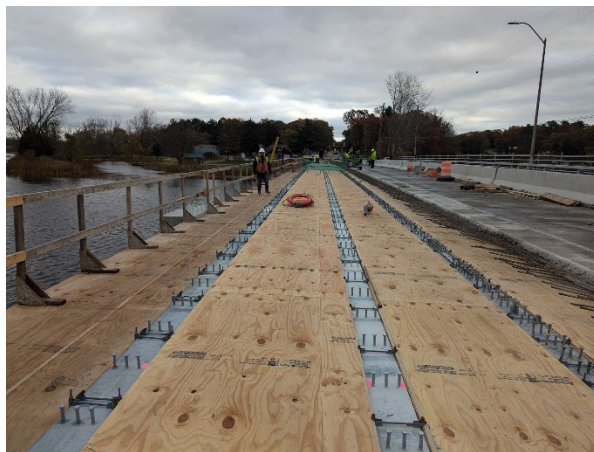
New bridge beams with wood concrete forms
