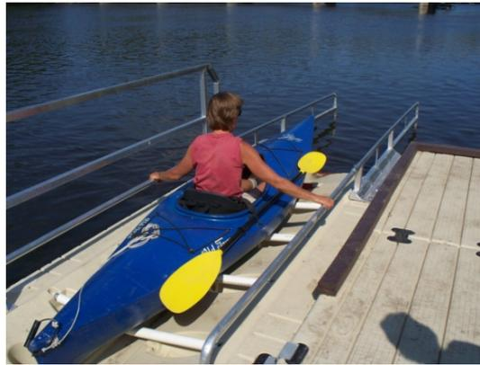
The roller system on the new barrier free canoe and kayak launch at Eastmanville Bayou provides a safe and stable means of launching for people of all abilities.
