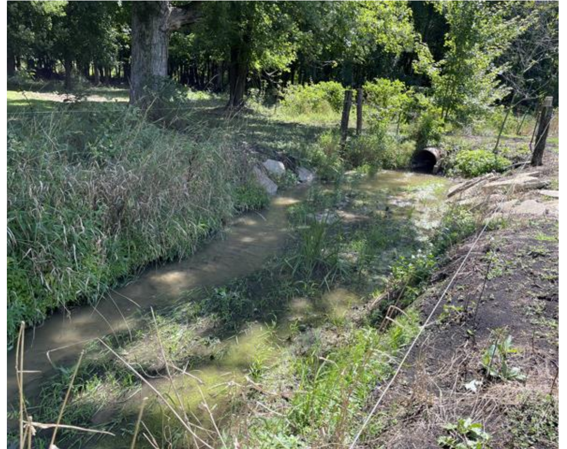
Private Crossing at Sta 16+50
