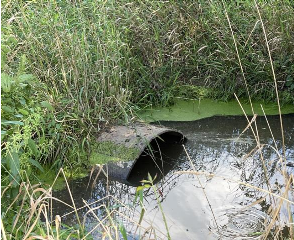
Ottogan St Culvert, partially submerged
