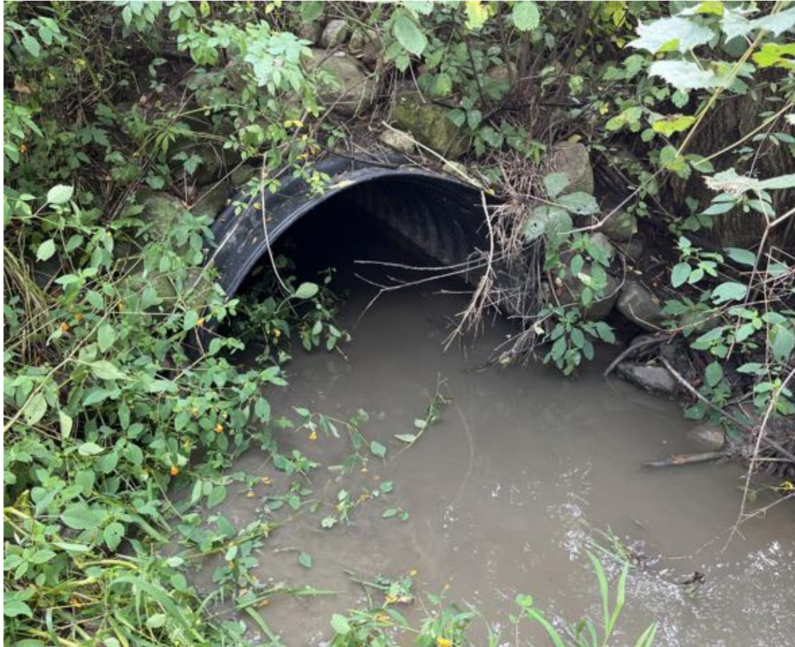
Private Crossing at Sta 21+25
