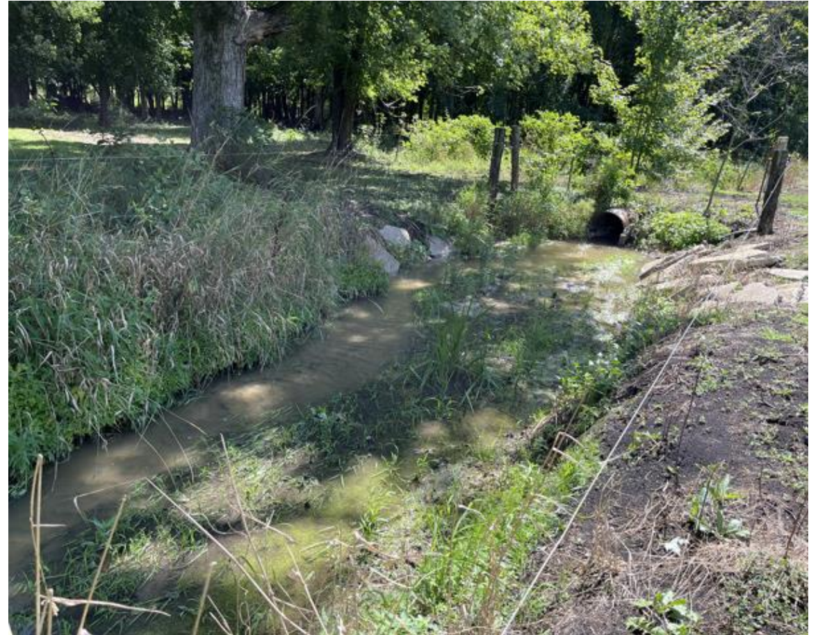
Mid-channel bars Sta 16+50 in dredged stretch
