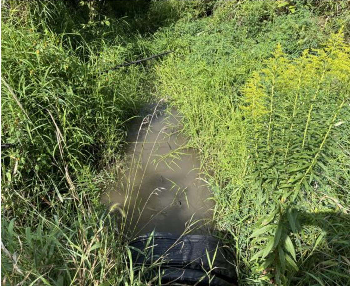
Private Crossing at Sta 58+25, Looking Upstream
