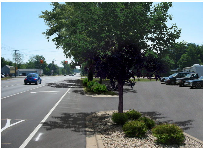
Exhibit 1-1b Same parcel with access management techniques (Landscaping and access point definition, must comply with all traffic and safety standards)
