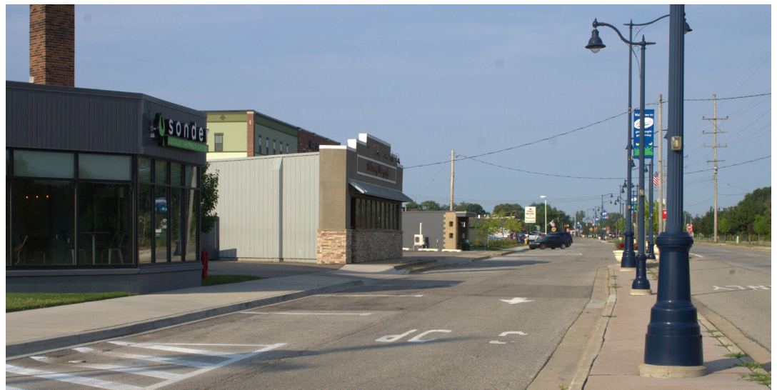
Service Street/Chicago Drive looking west.
