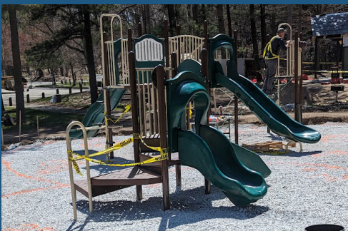
A new playground has been replaced and relocated.
