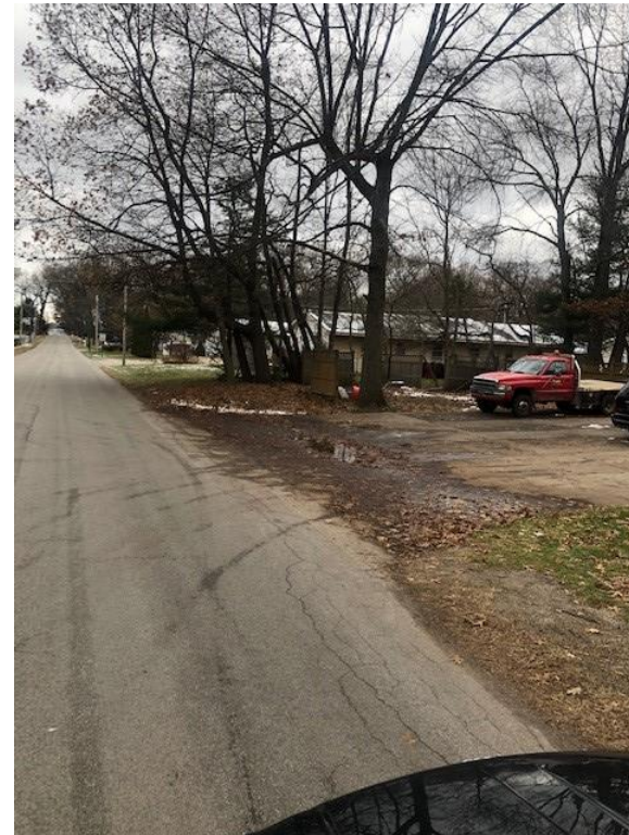
Standing water in the driveway approach along Beach Drive
