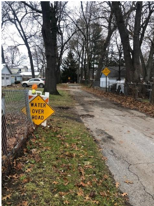
Standing water on Lane Avenue north of Railroad Avenue looking north
