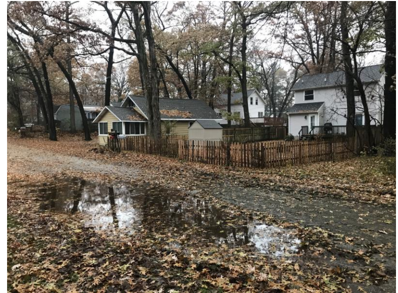
Standing water along the east side and saturated lawns on the west side of Oak St between Pine St and Cherry St
