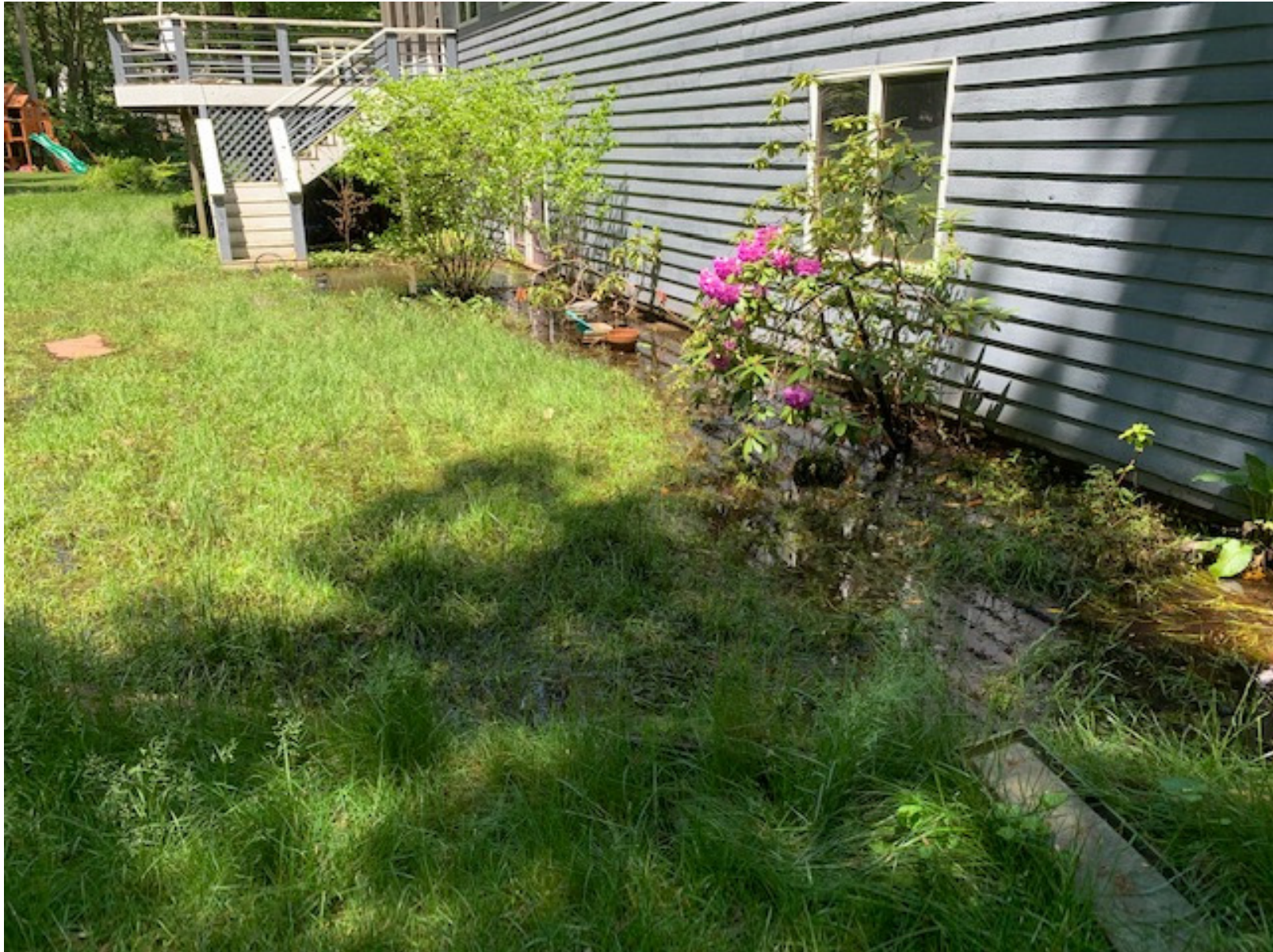
Retention Pond/Easement Area #5 – Ponding at back of 18702 Aztec Drive (6/10/19)
