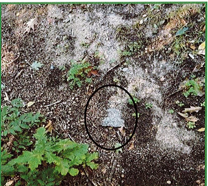
Culvert filled with sediment
