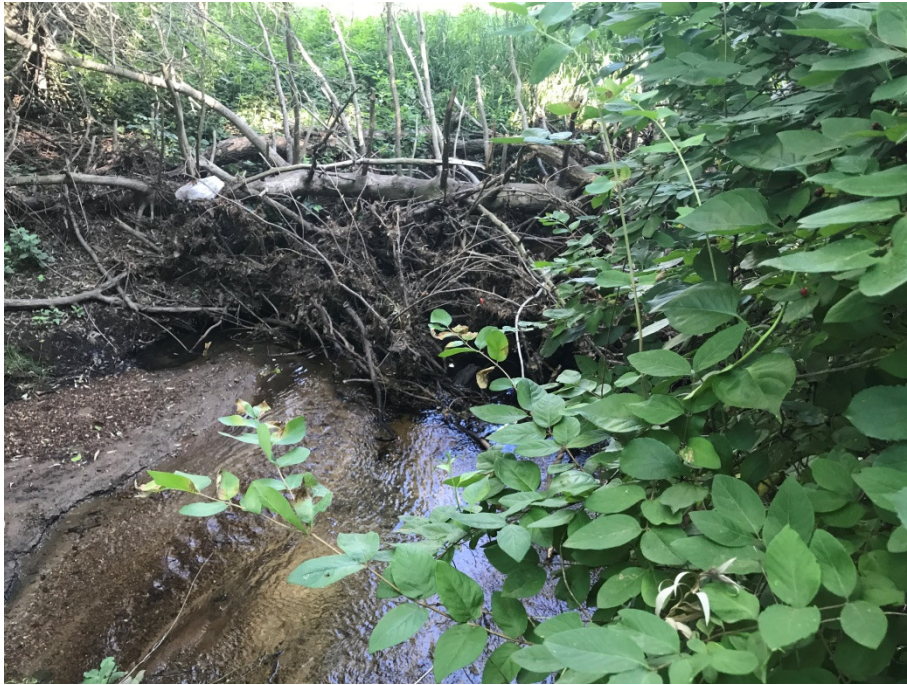
Log jam in drain near southwestern edge of soccer field fence
