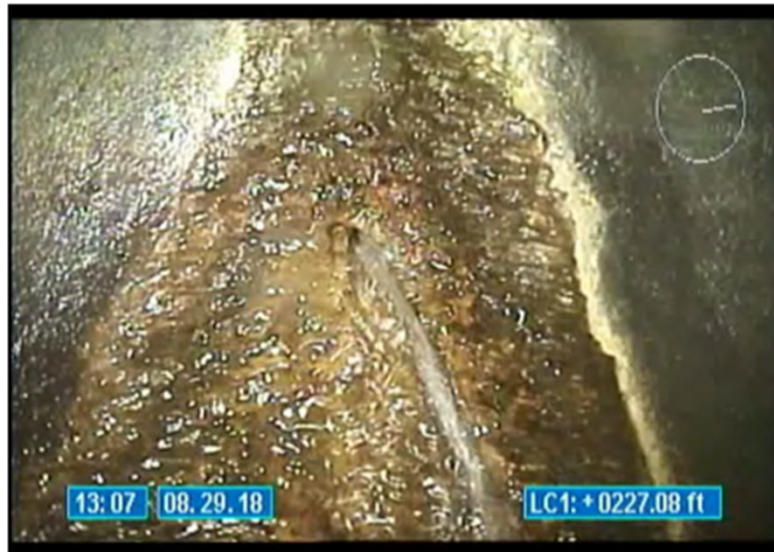
Infiltration through joints (photo on the left) and infiltration through a hole (photo on the right) in the 36 inch storm sewer.
