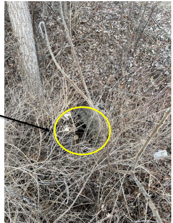
Culvert opening on east end of open drain, obstructed by debris.
