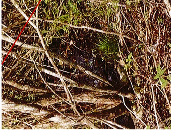
No established drainage channel to allow proper flow just west of Lost Creek Lane.
