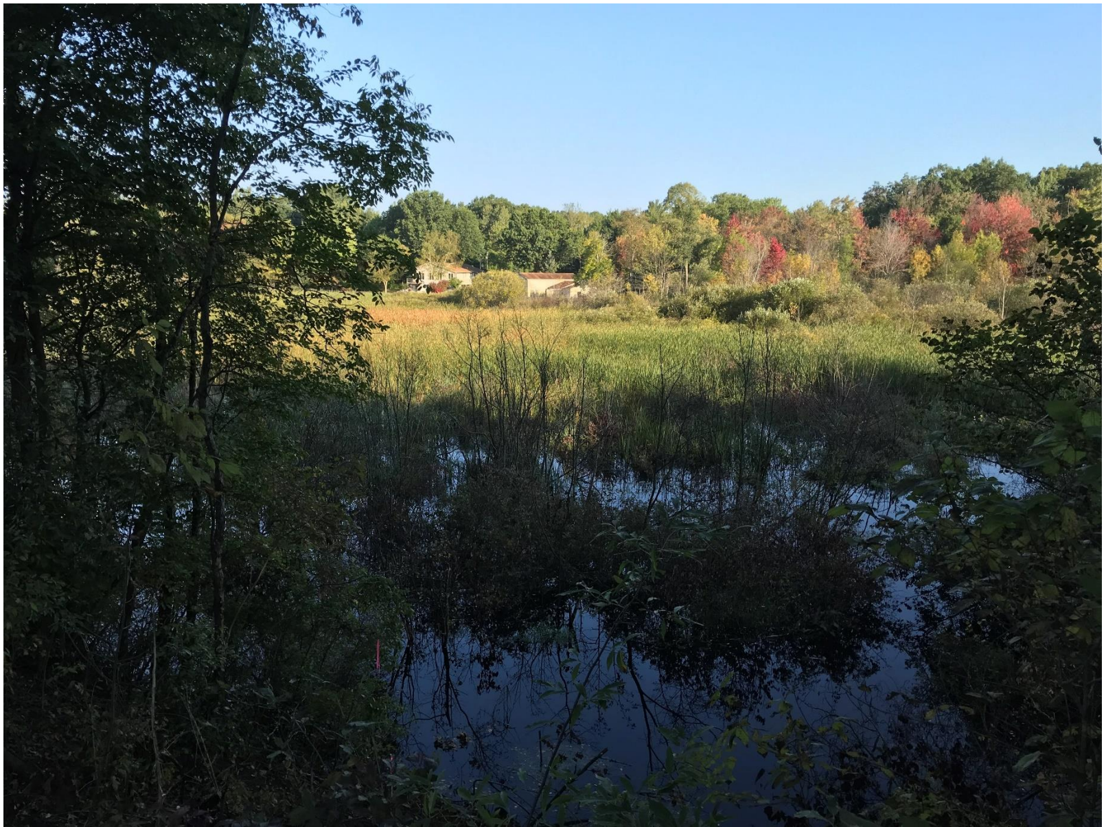
Flooding of wetlands upstream of culvert.
